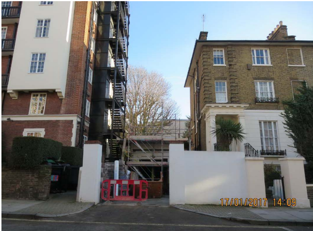
Site in view from Hill Road. 'Garage studio' under construction (January 2017).
